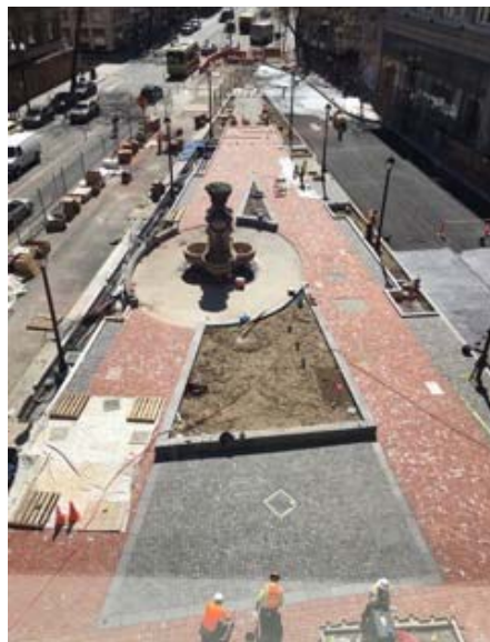
Latham Square Plaza Work
