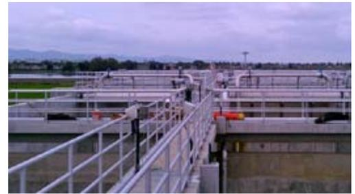
CMU block building, UV/Effluent pump station, and the solids handling building. Many of the structural features are already complete, and the construction contractors are busy this summer with installation, startup, testing, and training associated with the equipment at these facilities.
