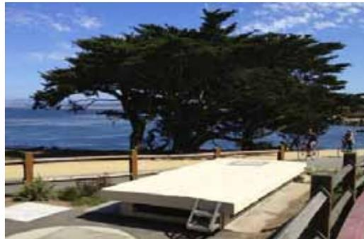
Our featured project for this edition is the Reconstruction of Wastewater Pump Station 12 in Pacific Grove. As a member of a team led by Psomas, TJCAA designed the structural elements of this upgrade, which included replacement of an above-grade emergency generator with a below-grade unit. The design featured a precast vault sited next to the existing vault, and left the existing pumping station in place.
