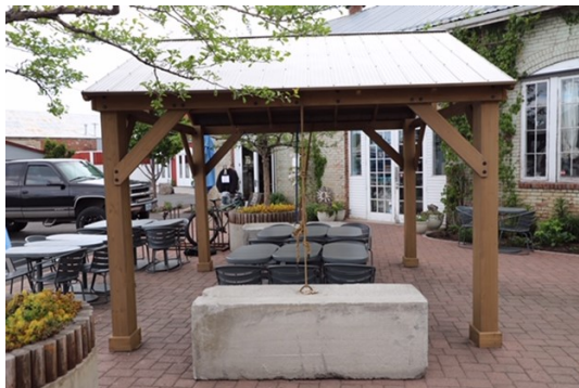
Contractor retrofit for "engineered" structure Photo - Rick Cavanagh
