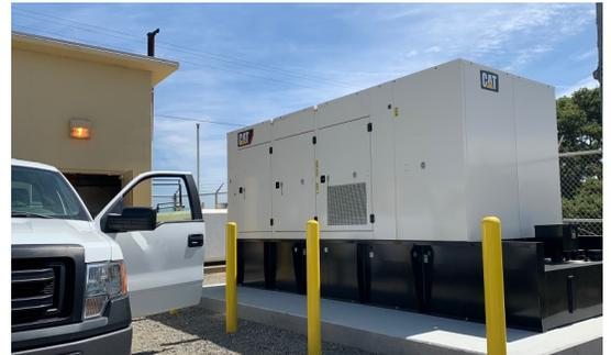
Backup power systems are generally designed for short-term use. Depending on demand and how "short-term" the use may be, a UPS (uninterruptible power supply) or generator may be desirable.
