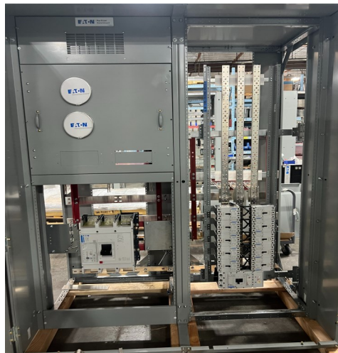
Switchboard Under Construction
